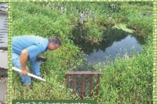
Goal 7: Culvert Inventory
