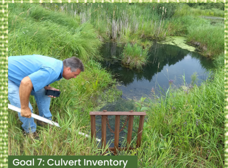
Goal 7: Culvert Inventory
