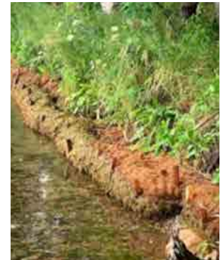
1 Watershed 1 Plan — Before & After on a private landowner's shoreline on Lower Hay Lake in Pine River, MN. Site visit conducted by CW SWCD & Prairie Restoration installed the coir logs & plants.
